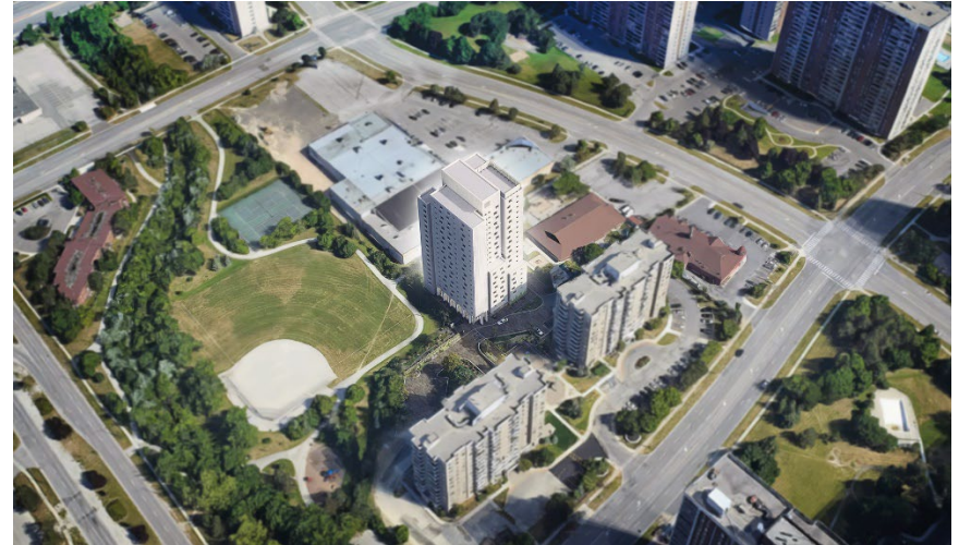
Chelsea Gardens-Net Zero Emissions New Construction affordable housing
