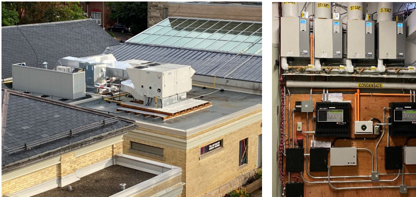
PAMA HVAC Replacement Project
