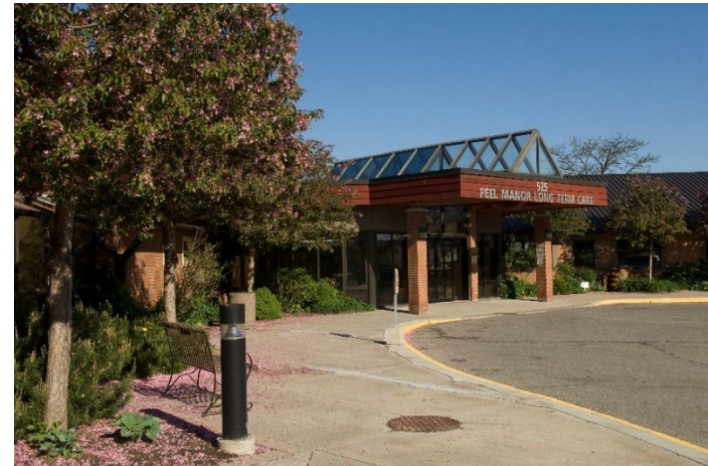
Peel Manor long term care home: currently being redeveloped to the new Seniors Health and Wellness Village
