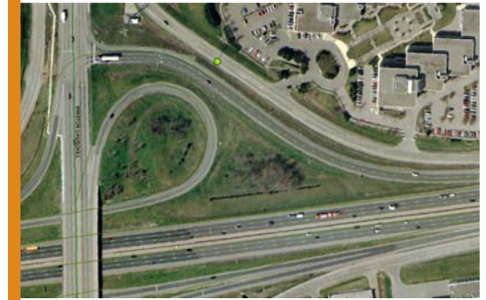
Highway 401 & Winston Churchill Blvd. Interchange, Mississauga
